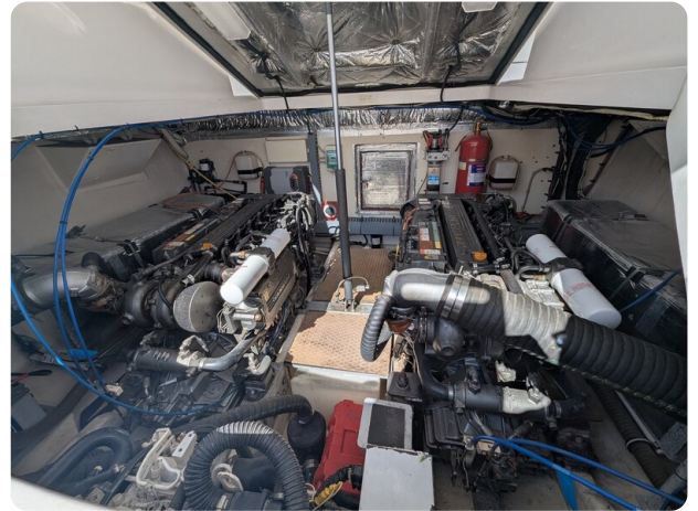
Luhrs 36 Open engine room
