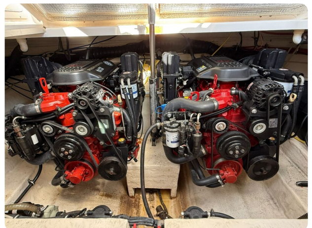
CHAPARRAL SIGNATURE 310 Engine room
